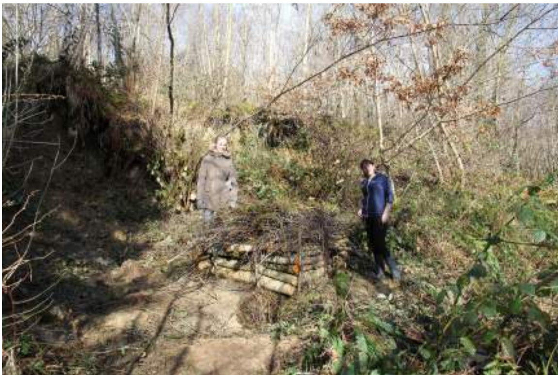
Figure 8 Finished log pile (logs were sourced from nearby tree limbs cut down by trained RSS participants)
