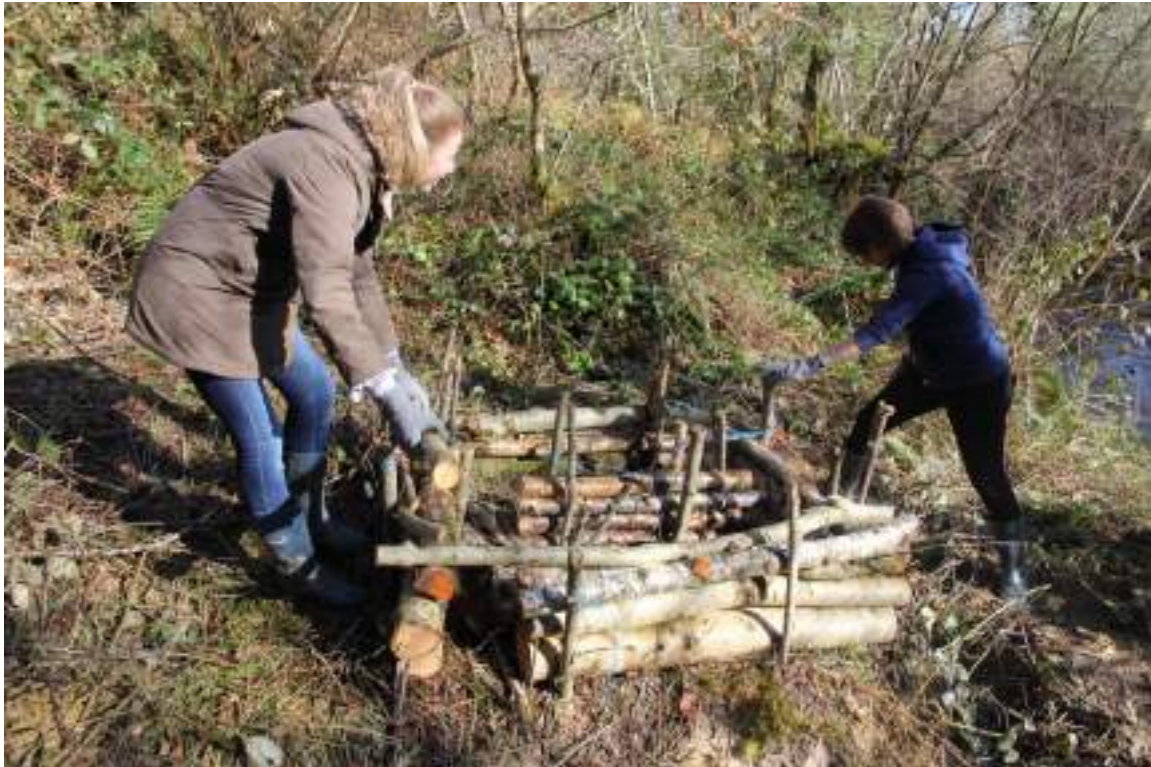
Figure 7 Volunteers constructing a log pile holt along the banks of the Dalua (Liscongill)
