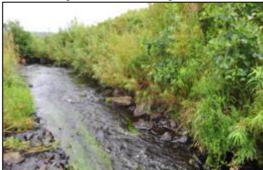
Willow wattling work on the Allow River (Image: Ruairí Ó Conchúir)
