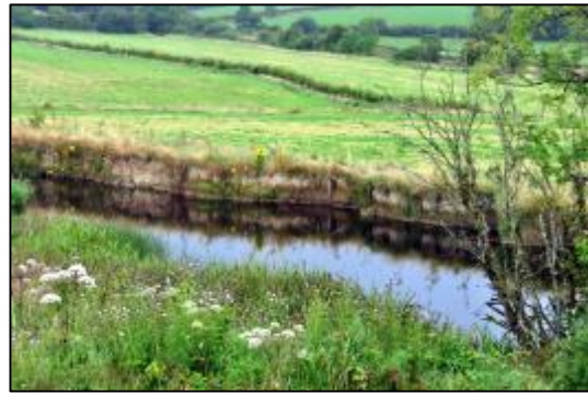
Work to stabilise bank erosion, Allow River (Image: Ruairí Ó Conchúir)
