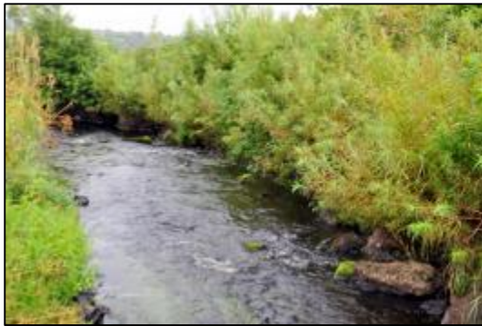
Willow wattling work on the Allow River (Image: Ruairí Ó Conchúir)
